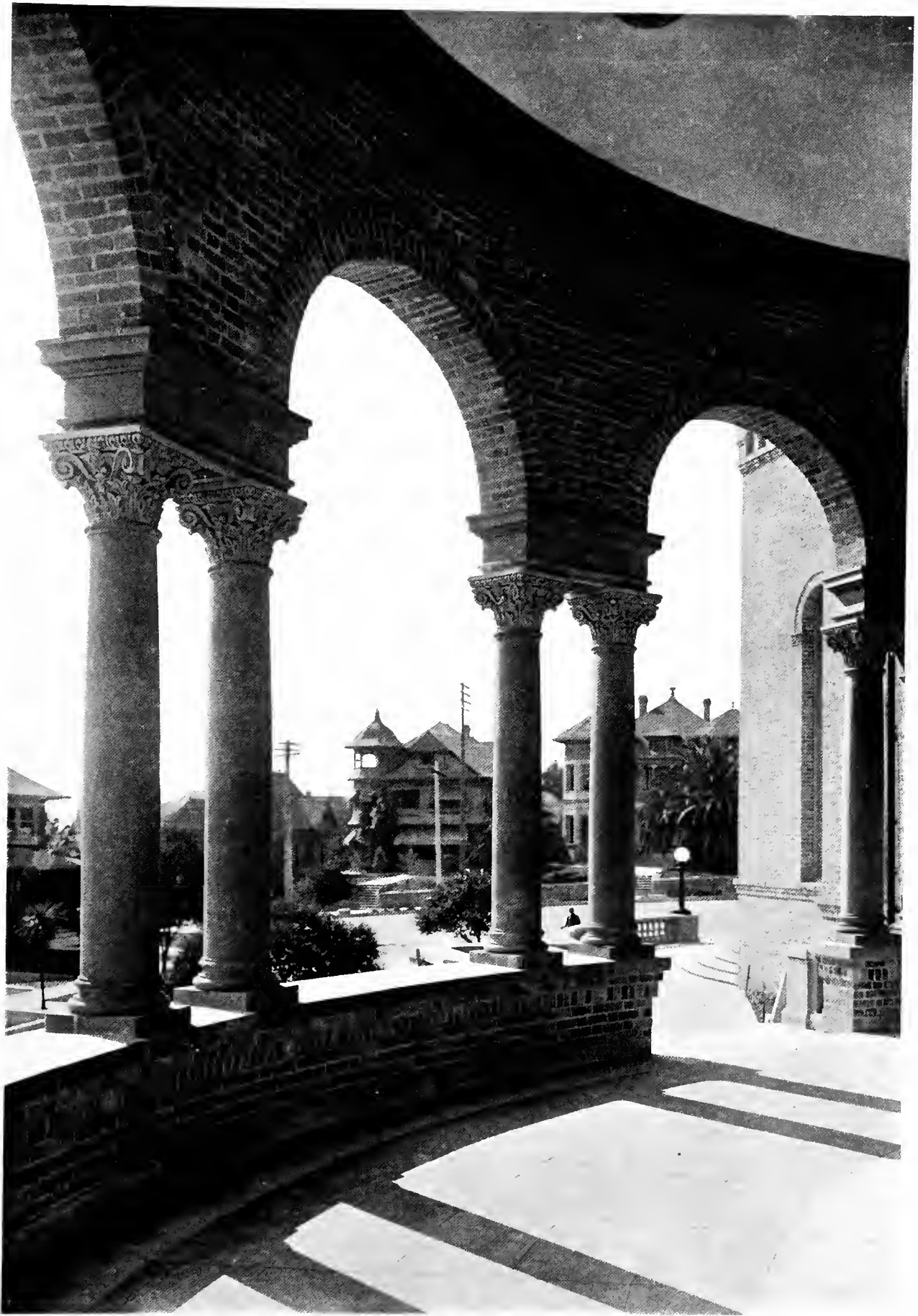
DETAIL OF LOGGIA
